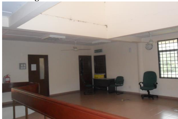
Figure-2. Interior Condition of TSM
