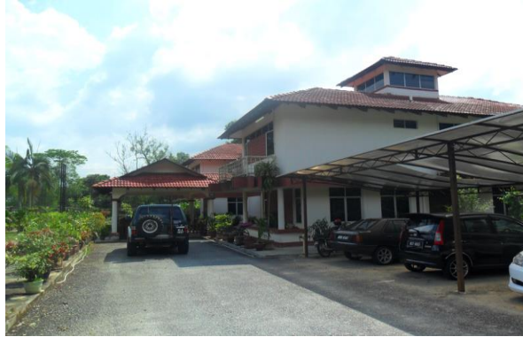
Figure-1. Tapak Semaian Mantin (TSM) office building and its surroundings
