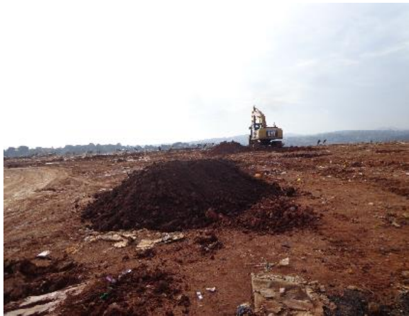
Prospector UAP 367L Strengthening soft areas within Southern Tipping Front 23 rd September 2013
